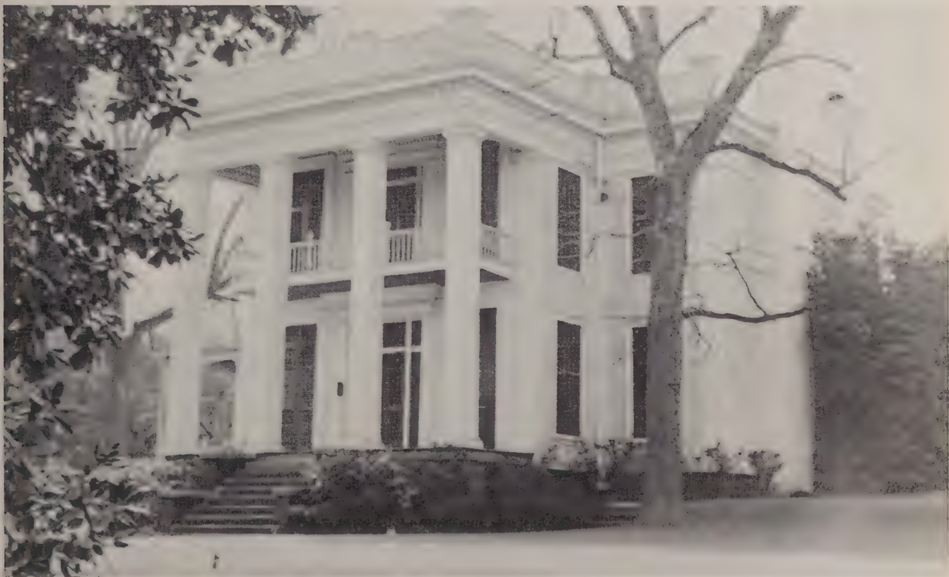
McBryde-Screws-Tyson home on Mildred Street at the head of Goldthwaite Street built in 1832 still being used by a descendant, and in excellent condition.
